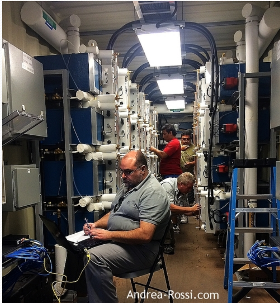
Assembling 1 MW unit 2014
